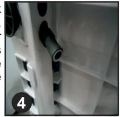
5. Place the tap supplied by the kit to close the remaining hose. Connect the new drain hose to the waste black water pipe.
